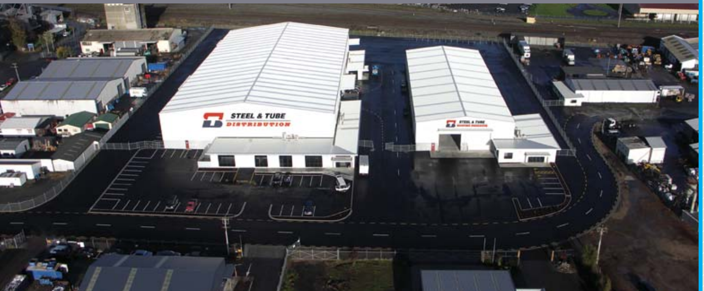
New premises for Distribution and Roofing in Hamilton
