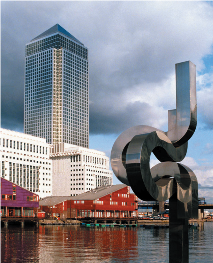
Photograph: Canary Wharf Tower, London's Docklands, built with structural steel and stainless steel cladding.
